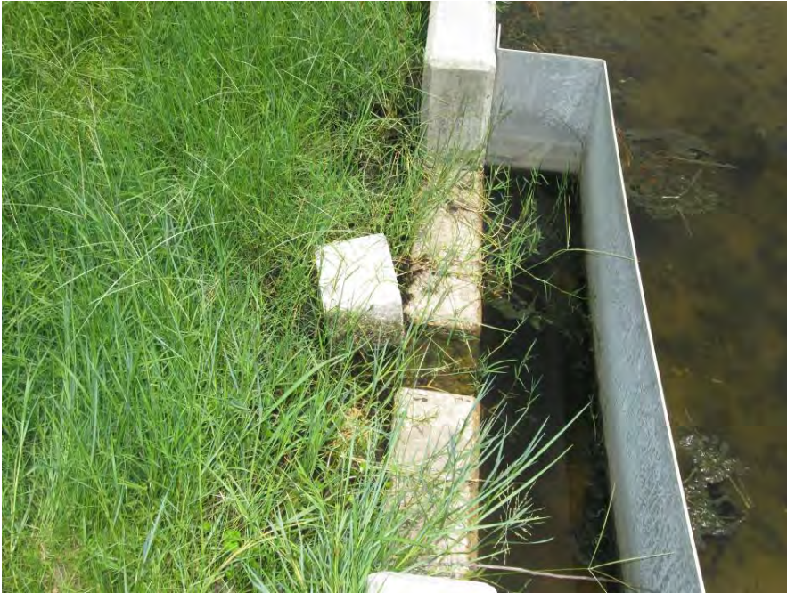
Site 5 – pond 35 – remove concrete block behind weir
