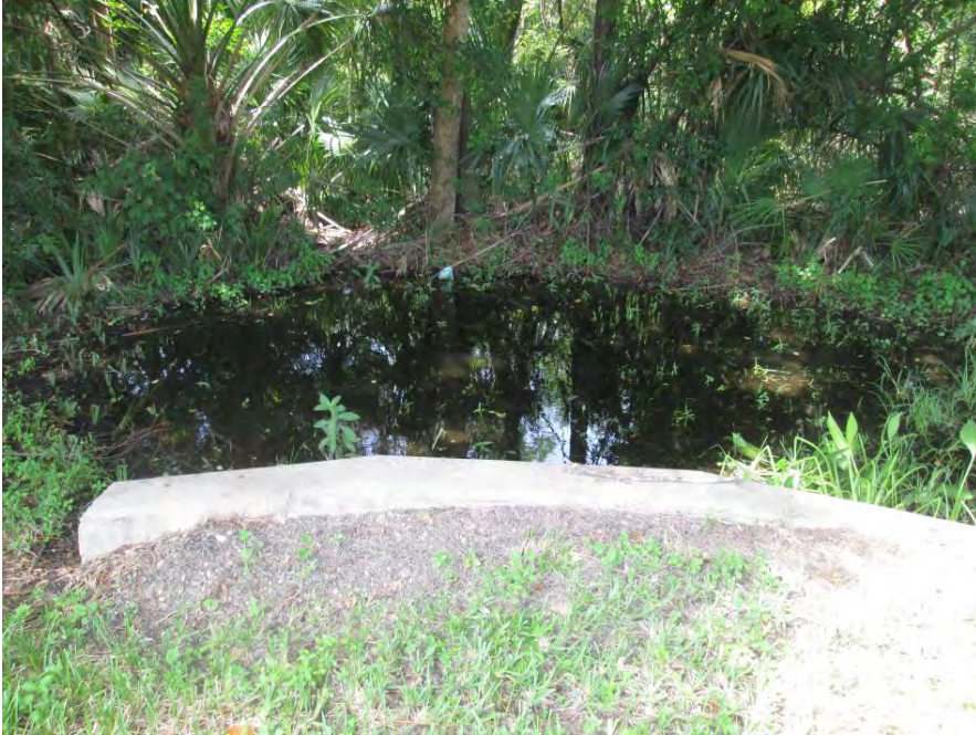
Site 13 – Tailfeather e/o Cormorant – debris & tree causing ponding
